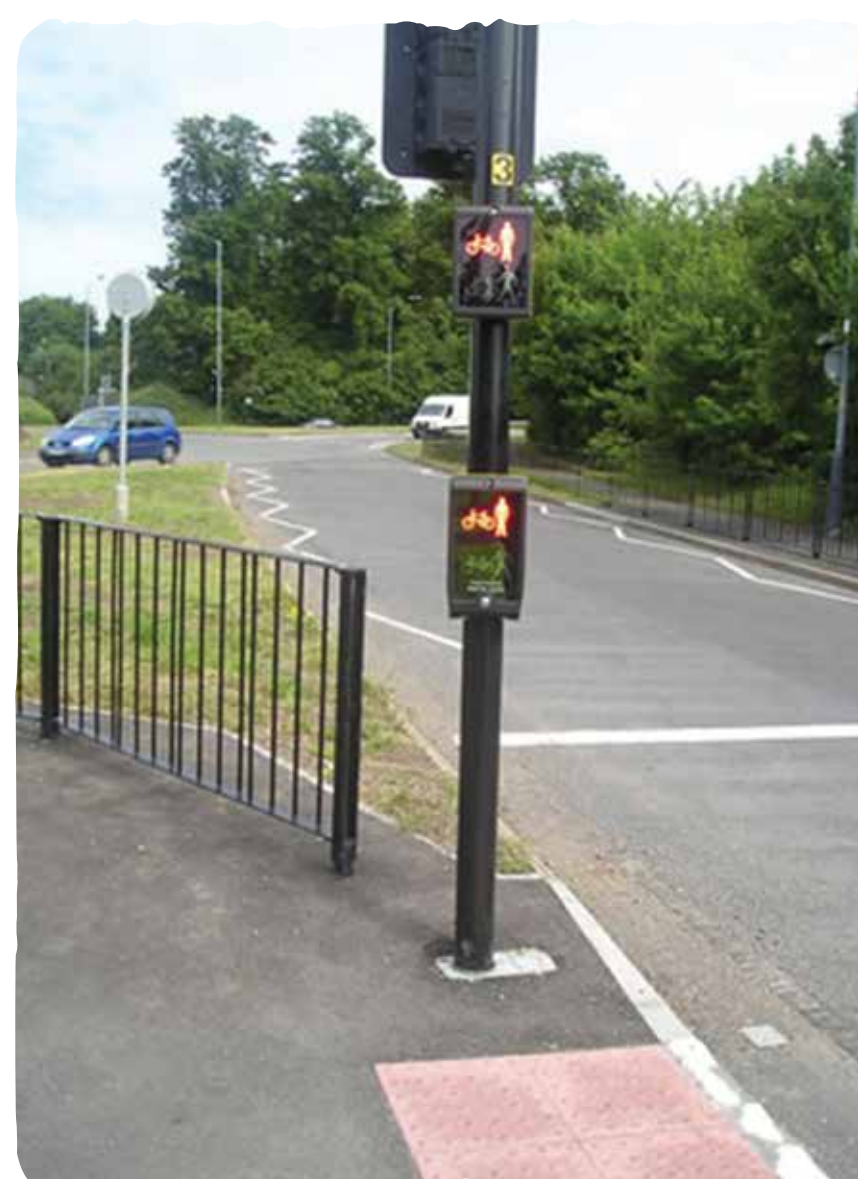
Toucan crossings will be installed to make crossing the road easier for pedestrians and cyclists
